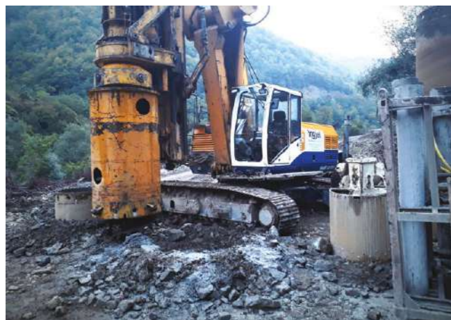
Izvedba armirano betonskih pilota promjera 1.200 mm u koritu rijeke u izrazito nepovoljnim slojevima tla (tvrda stijena) Construction of concrete piles with a diameter of 1,200 mm in the riverbed, in extremely unfavorable soil layers (hard rock)
