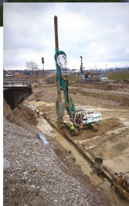
Izvedba armirano betonske i glinobetonske dijafragme Reinforced concrete and clay concrete diaphragm execution
