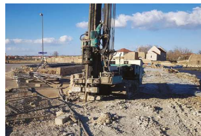
Gornji most - oštećeni most; izvedba mlazno injektiranih stupnjaka; bušilica nakon velikog nevremena Upper bridge - damaged bridge; jet-grouting columns execution; drilling machine after a major storm
