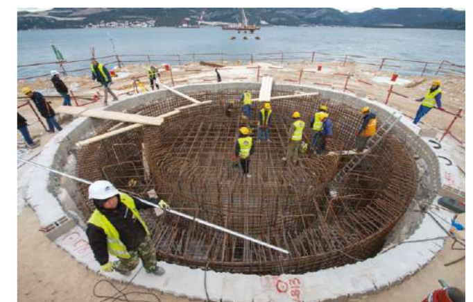
Građevinska jama od sekantnih pilota ispod razine mora i armirano betonski piloti temelja stupišta S13 Below-sea-level construction pit of secant piles and reinforced concrete piles for the S13 pier foundation
