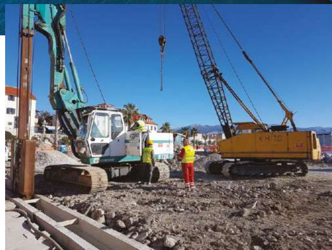
Iskop dijafragme upotrebom grajfera Diaphragm excavation using a greifer
