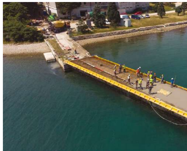
Betoniranje i asfaltiranje ploče mosta Bridge deck concrete and asphalt paving
