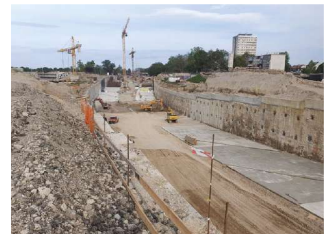
Uspješno izvedena zaštita građevinske jame podvožnjaka Successfully performed protection of the underpass construction pit
