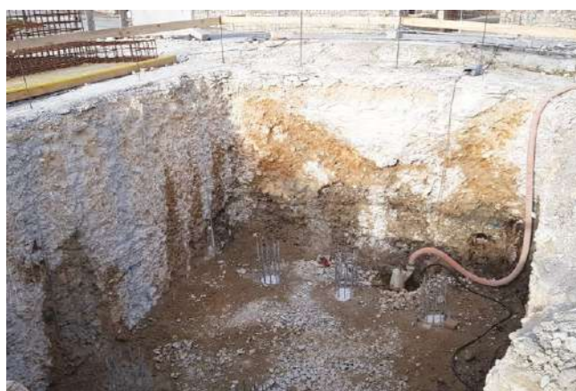
Donji most: Izvedba mlazno injektiranih stupnjaka s dvije bušilice, iskop građevinske jame te uspješno izvedena građevinska jama za rad u suhom Lower bridge: Jet-grouting columns execution with two drilling machines, excavation of a construction pit and successfully performed construction pit for dry work
