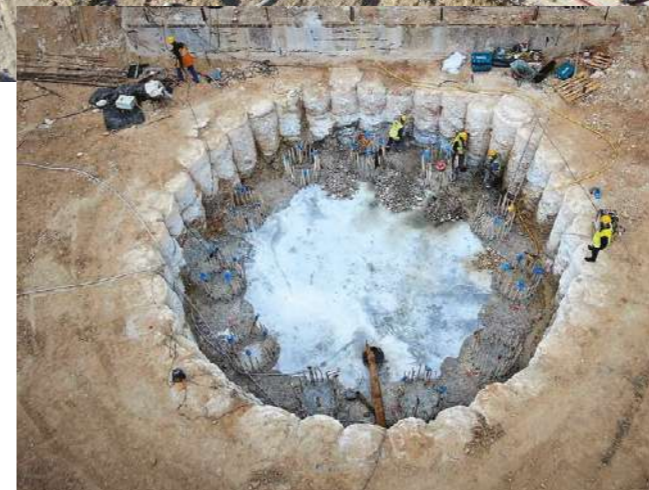
Građevinska jama od sekantnih pilota ispod razine mora i armirano betonski piloti temelja stupišta S13 Below-sea-level construction pit of secant piles and reinforced concrete piles for the S13 pier foundation
