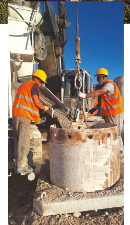
Ugradnja betona Concrete installation
