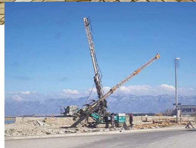
Gornji most: Izvedba mlazno injektiranih stupnjaka s dvije bušilice, povratna cementna suspenzija te uspješno izvedena građevinska jama za rad u suhom Upper bridge: Jet-grouting columns execution with two drilling machines, returned cement suspension and successfully performed construction pit for dry work
