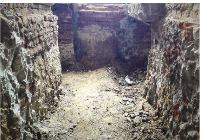
Above: Foundation strengthening and construction pit protection Below: Foundation strengthening and basement deepening
