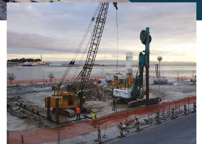
Izvedba dijafragme uz Trumbićevu obalu Diaphragm execution along the Trumbić coast
