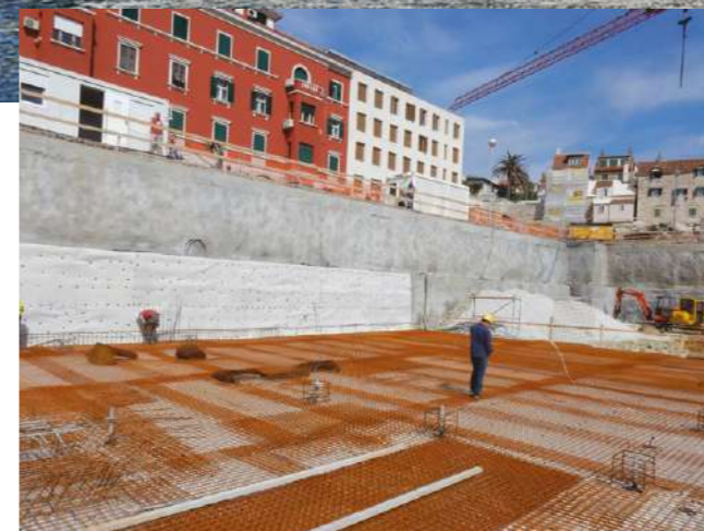
Uspješno izvedena građevinska jame za rad u suhome, 7 m ispod razine mora Successfully performed construction pit for dry work, 7 m below sea level
