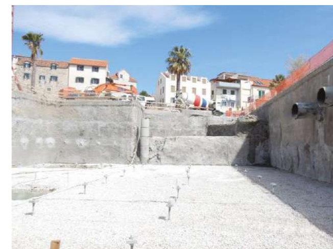
Uspješno izvedena građevinska jame za rad u suhome, 7 m ispod razine mora Successfully performed construction pit for dry work, 7 m below sea level
