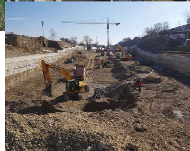
Uspješno izvedena zaštita građevinske jame podvožnjaka Successfully performed protection of the underpass construction pit
