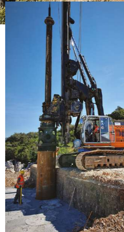
Izvedba bušotine promjera 1.500 mm Borehole execution with a diameter of 1,500 mm
