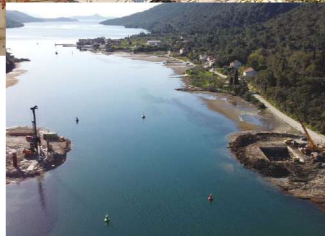
Izvedena građevinska jama ispod razine mora (sekantni piloti i čelične razupore) Performed construction pit below sea level (secant piles and steel struts)
