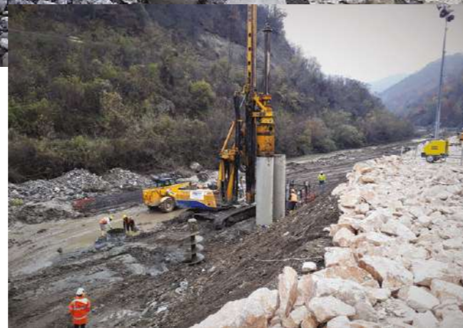
Izvedba armirano betonskih pilota promjera 1.200 mm u koritu rijeke u izrazito nepovoljnim slojevima tla (tvrda stijena) Construction of concrete piles with a diameter of 1,200 mm in the riverbed, in extremely unfavorable soil layers (hard rock)
