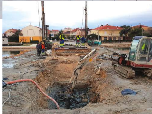
Donji most: Izvedba mlazno injektiranih stupnjaka s dvije bušilice, iskop građevinske jame te uspješno izvedena građevinska jama za rad u suhom Lower bridge: Jet-grouting columns execution with two drilling machines, excavation of a construction pit and successfully performed construction pit for dry work
