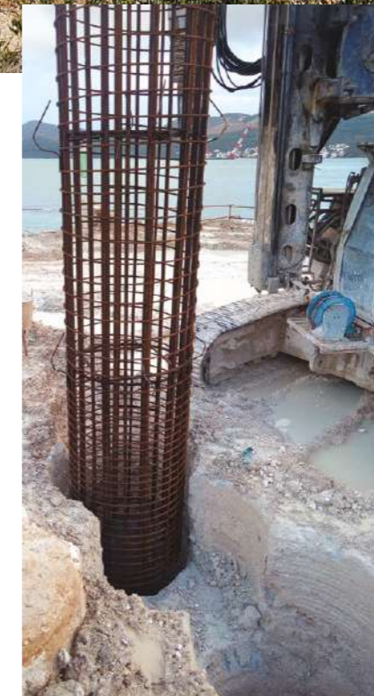
Ugradnja armaturnog koša Reinforcement cage installation
